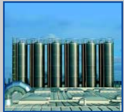
Pressure vessel construction
